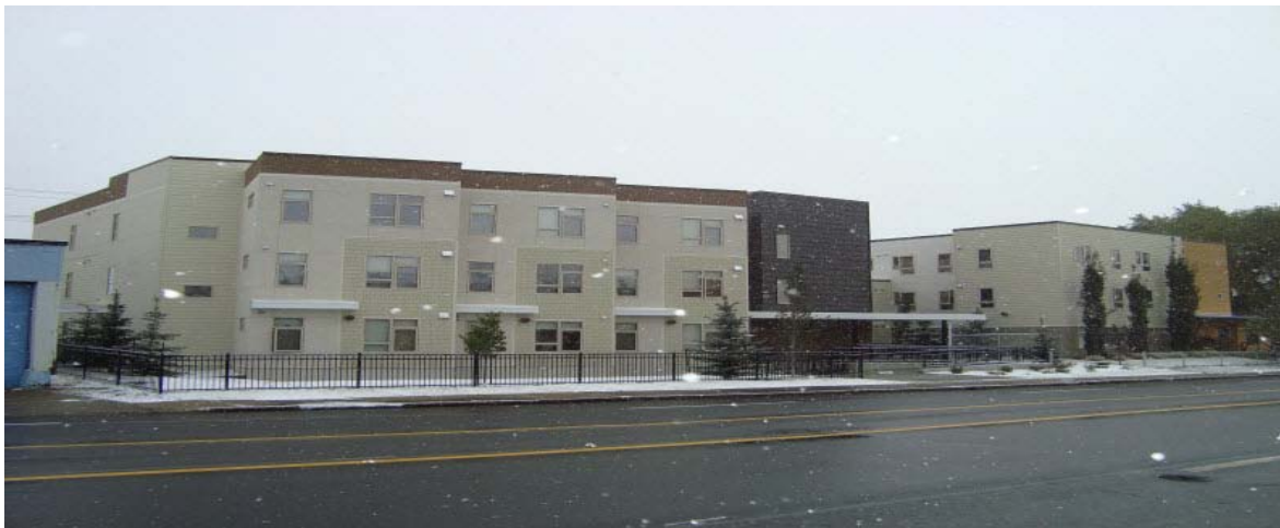
Alliance Manor Apartments
